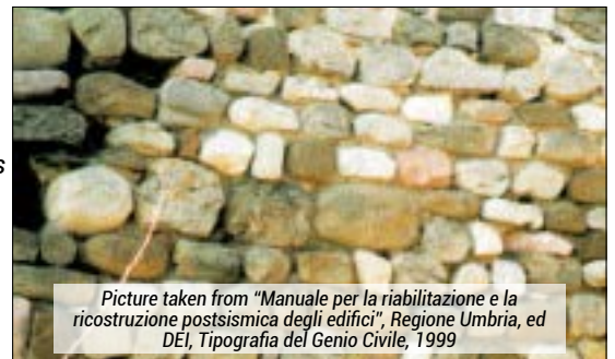
Assisi (PG): various types of pebbles with regular layout
