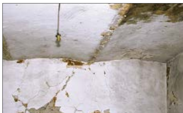
Floor with iron beams and shallow arch vaults
