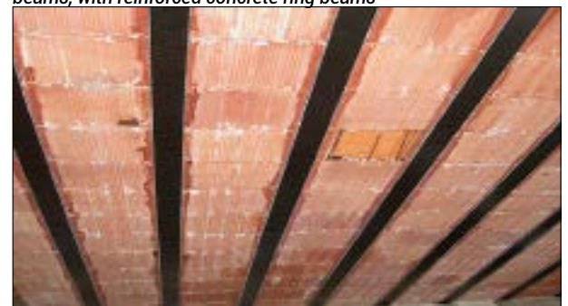
Floor made of iron beams supporting hollow clay tiles
