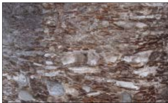
Alia (PA): irregular masonry with flat tiles and limestone
