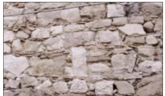
Cast. dei Sauri (FG): Rubble stone masonry with brick courses
