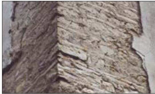
Benevento: rubble stone masonry with brick courses
