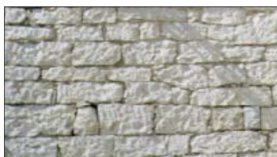
Cerchiara (CS): semi-dressed calcareous stone
