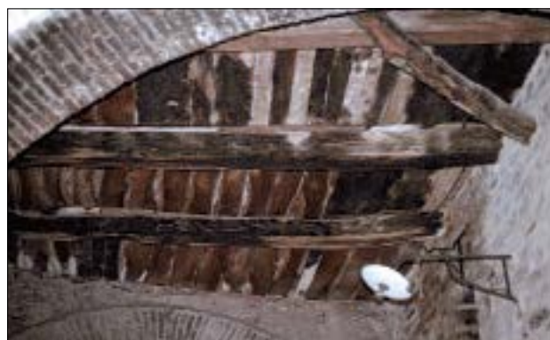
Wooden floor with wooden planks in a single direction
