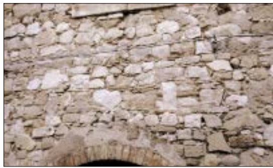
San Angelo Limosano (CB): rubble stone with irregular layout
