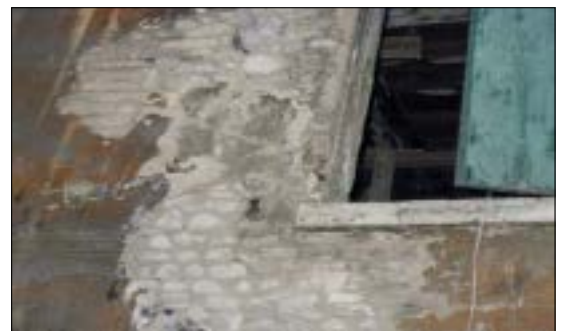
Sassuolo (MO): pebbles and bricks
